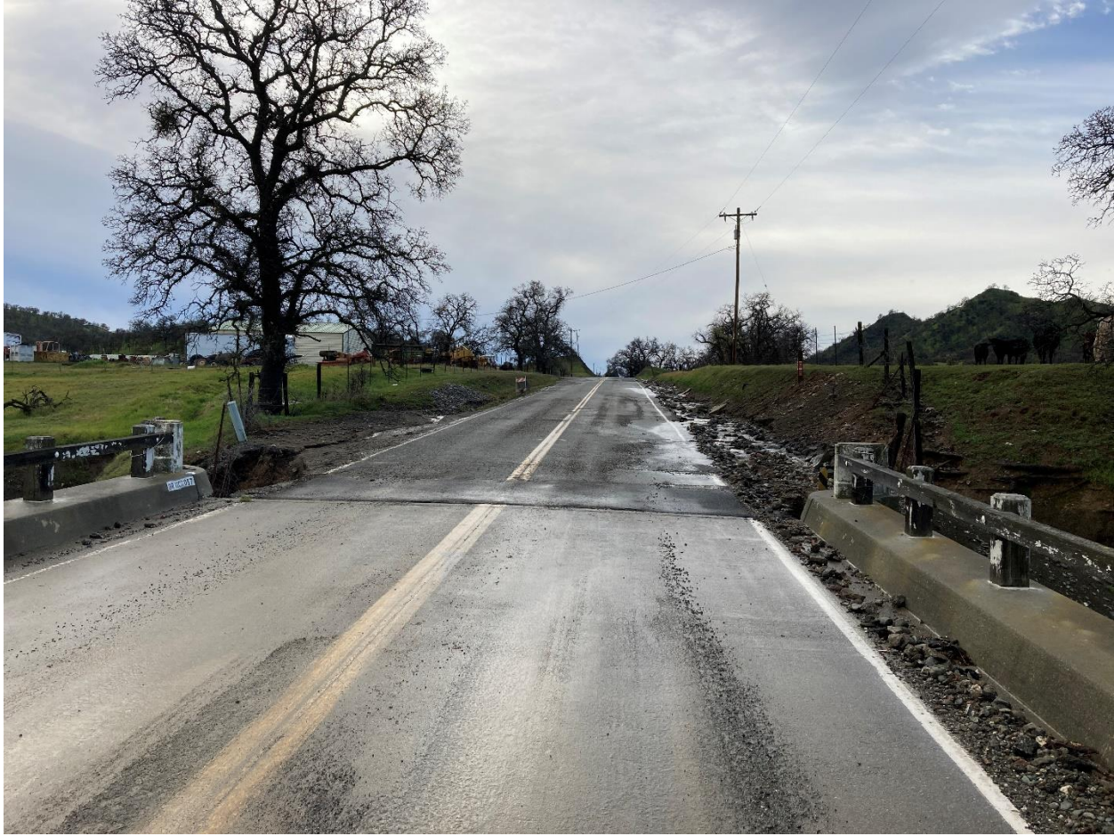
Figure 2 - BRIDGE 11C0057 LOOKING SOUTH
