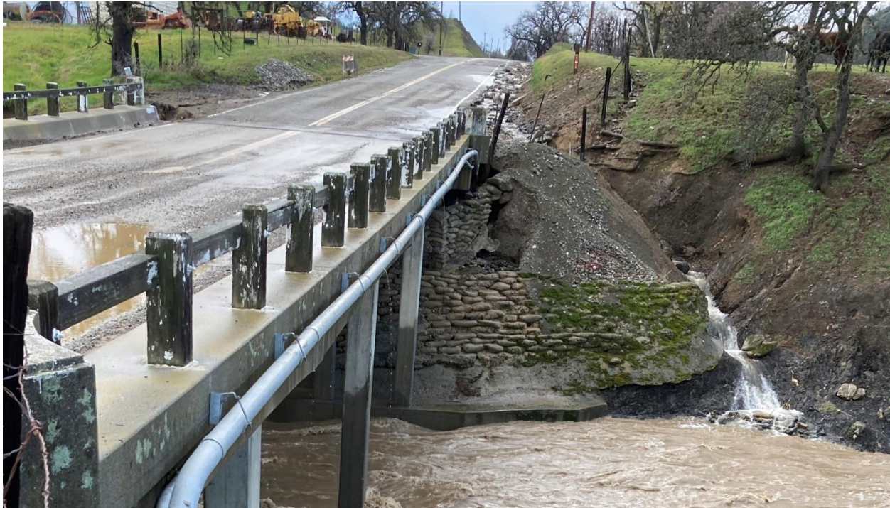
Figure 3 - BRIDGE 11C0057 LOOKING SOUTH
