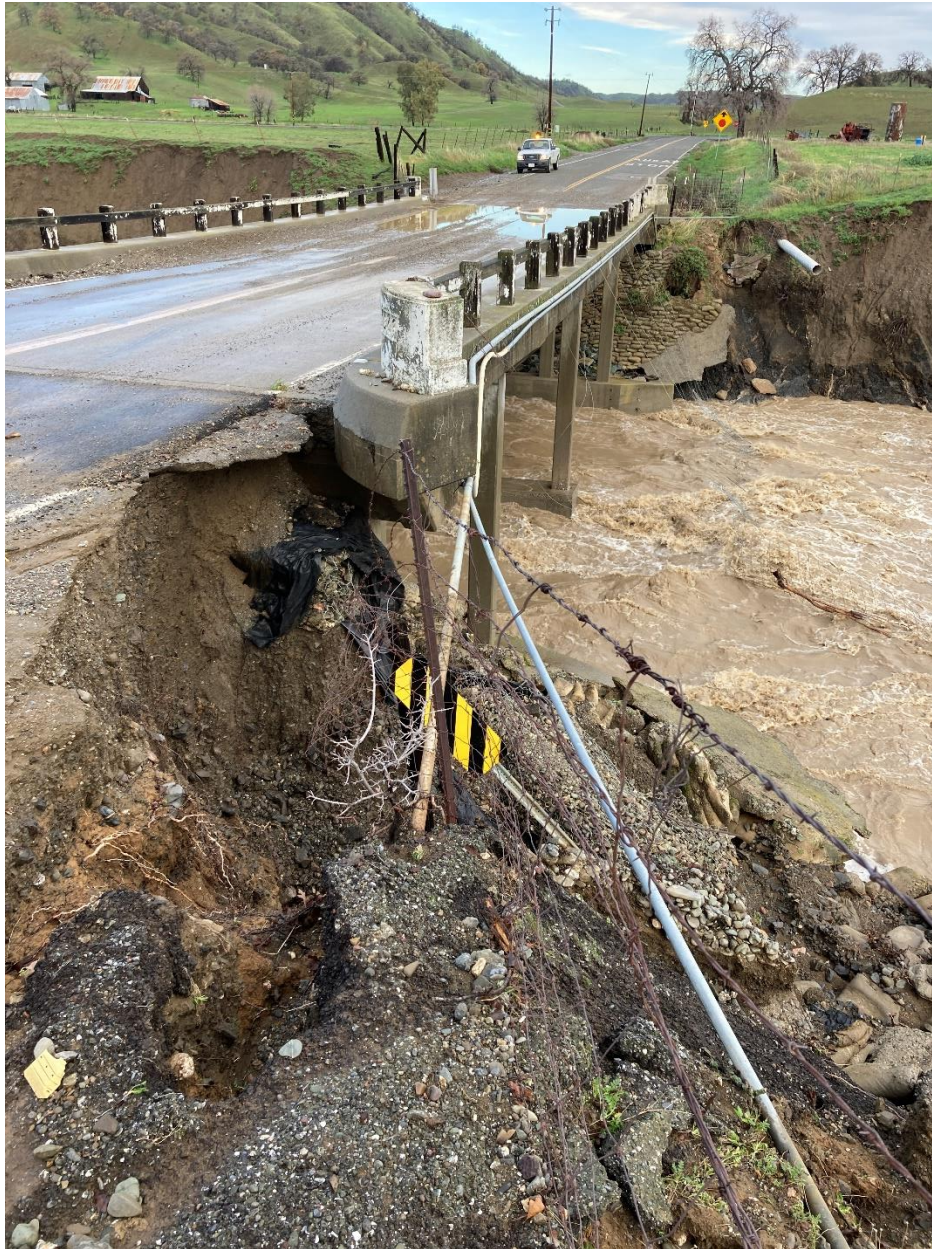
Figure 4 - BRIDGE 11C0057 LOOKING NORTH
